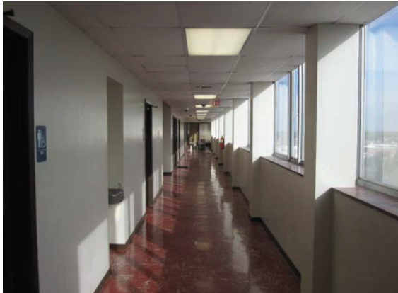
The corridors at the third, fourth and fifth floors (pictured), with original resilient tile flooring, plaster walls and ribbon windows.
