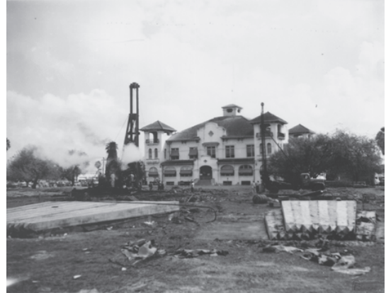
Construction progress photo, 1952. Image: Museum of South Texas History, 1991.37.03a.I.GovtBldgs.courthse12.
