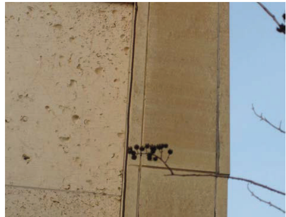
Some of the dolomitic limestone panels have been re-attached with surface mounted fasteners, such as the unit at the far right.
