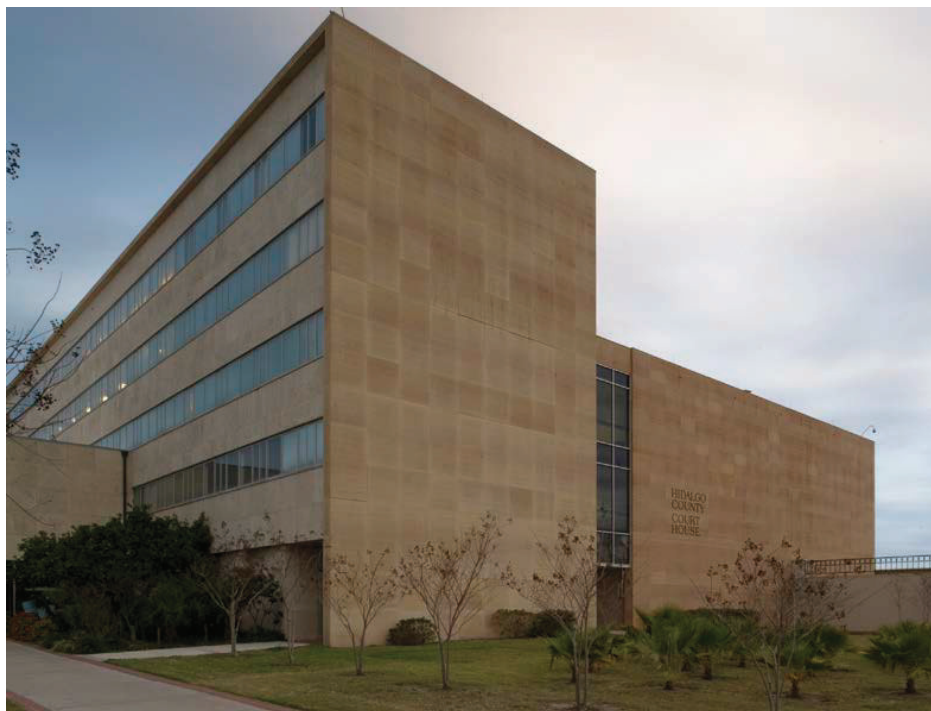
View of the original 1954 courthouse, on the left, and the 1980 addition, on the right, looking northwest, February 20, 2009. The sally port, added in 2006, shows at the far right. Image: © Capitolshots Photography.
