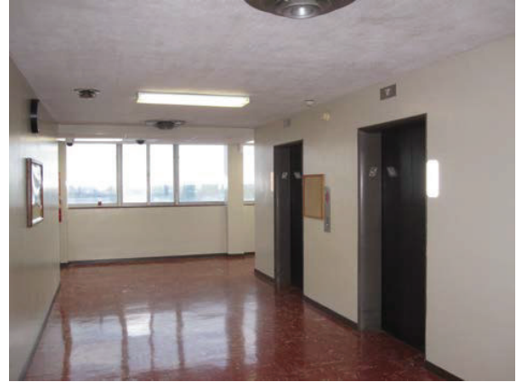
The fifth floor elevator lobby, with original plaster ceiling. A lay-in, acoustic tile ceiling has been added in the corridor, beyond.
