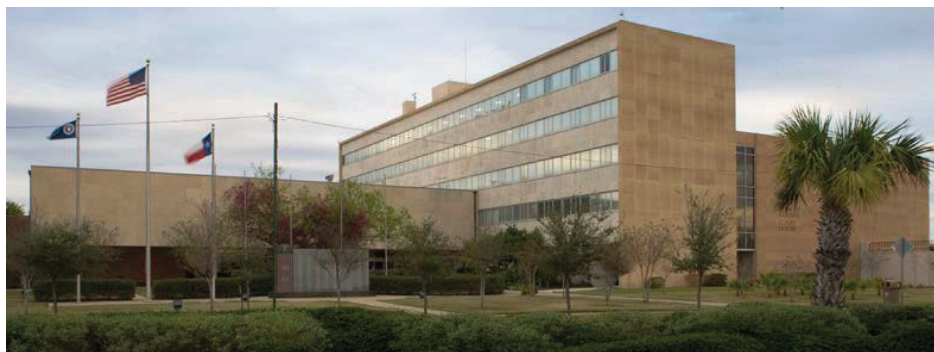
View of the original 1954 courthouse, on the left, and the 1980 addition, on the right, looking northwest, February 20, 2009. The sally port, added in 2006, shows at the far right. Image: © Capitolshots Photography.
