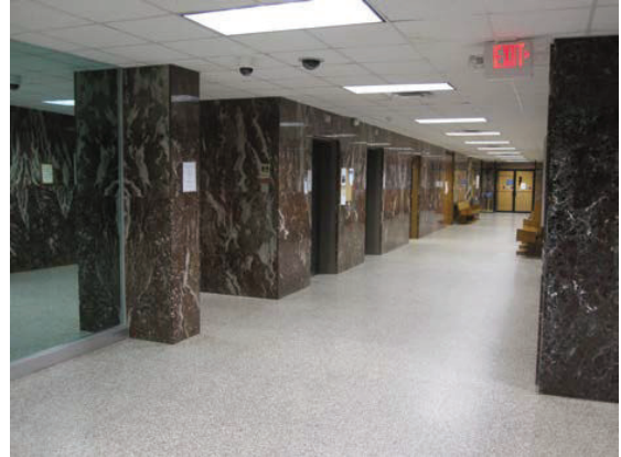
The second floor corridor, with original terrazzo flooring and marble wall panels, is furnished with original benches.
