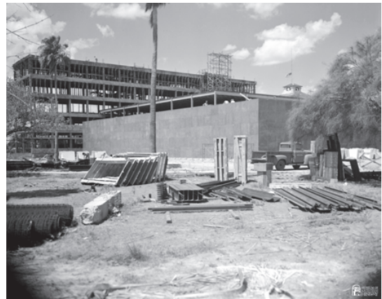
Construction progress photo, 1953. Image: Museum of South Texas History, 1991.37.03a.I.GovtBldgs.courthse20.
