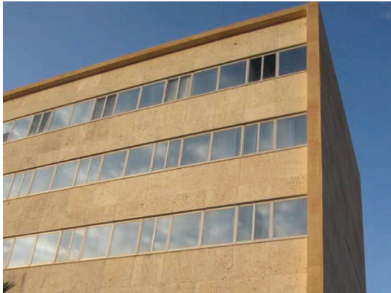
South elevation, showing shell limestone at left and dolomitic limestone at right and ribbon windows.
