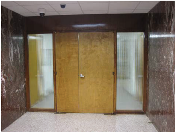
Terrazzo floor, marble wall paneling and wood slab door with ribbed glass sidelites at the second floor.
