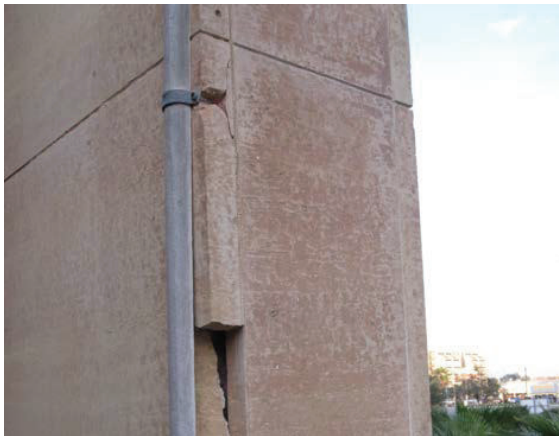
Cracked, damaged stone veneer, due to expansion of metal fasteners in the stone.
