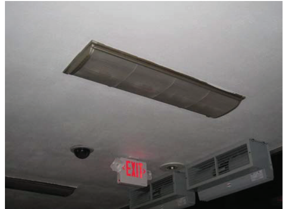
An original semi-recessed fluorescent light fixture in the plaster ceiling of the first floor entry lobby.
