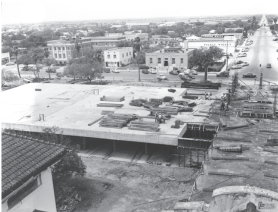
Construction progress photo, 1953. Image: Museum of South Texas History, 1991.37.03a.GovtBldgs.HCC (i).
