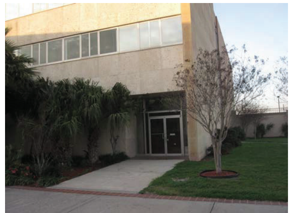
South elevation, showing non-original exterior doors. The 1980 addition and 2006 sally port show at the far right.
