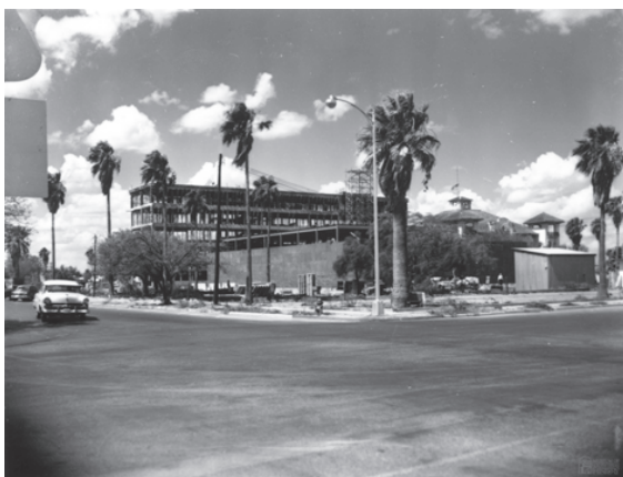
Construction progress photo, 1953. Image: Museum of South Texas History, 1991.37.03a.I.GovtBldgs.courthse14.
