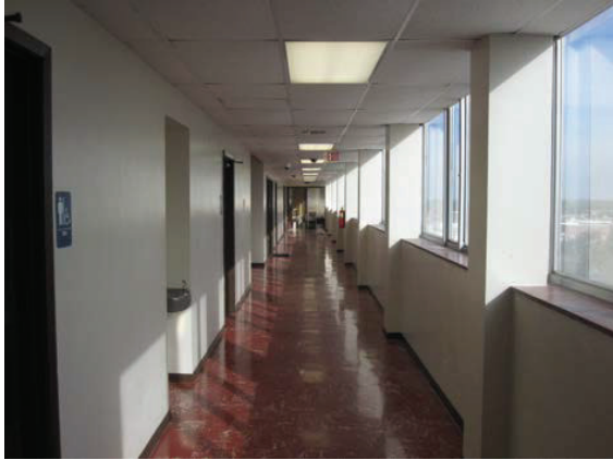
The south corridor at the fifth floor, showing resilient flooring, plaster walls and ribbon windows.
