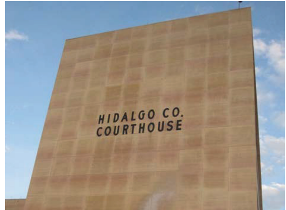
View of west elevation of the original tower, showing the distinctive dolomitic limestone veneer. (The signage is not original.)
