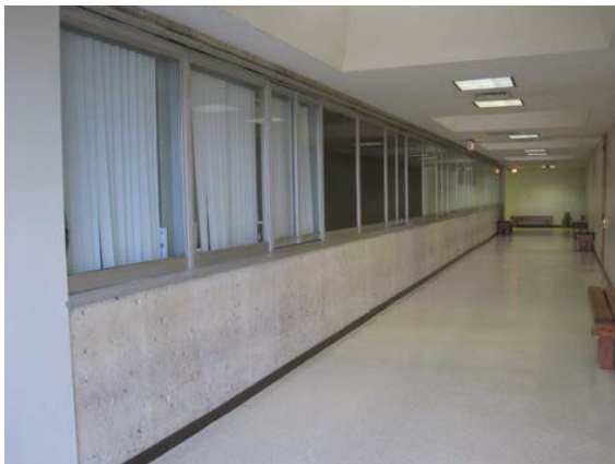
Original exterior ribbon windows remain on the second and third floors, enclosed in the corridors of the 1980 addition.
